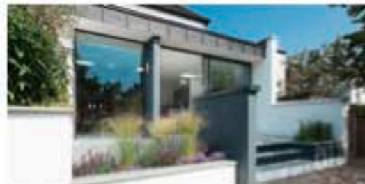
A highly innovative single-storey modern extension to a 3-bedroom...
